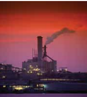
Sample and Instrumentation Filtration
