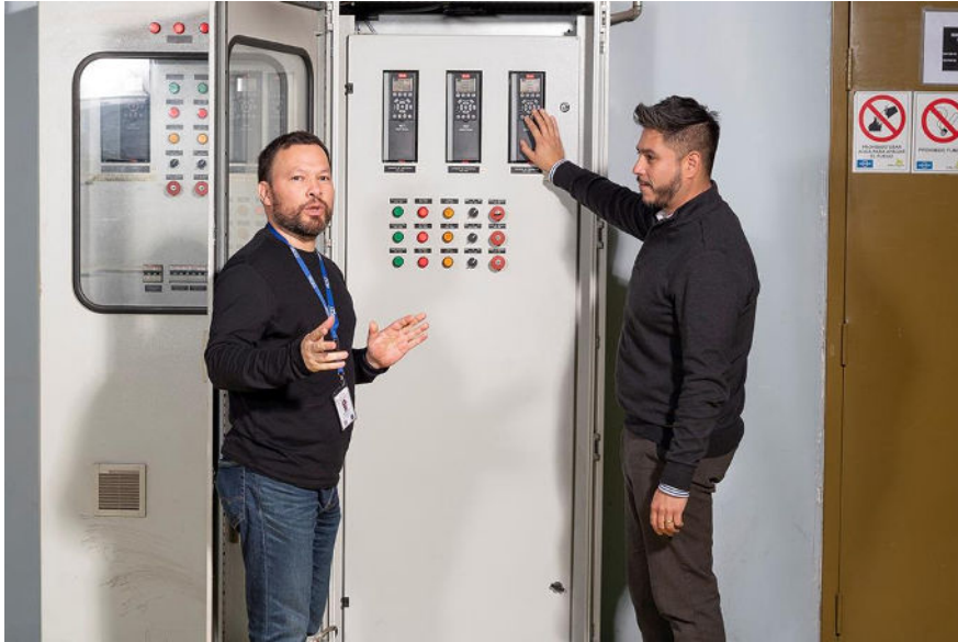
The VLT® drives are all located in the basement. In the photo from left: Maintenance Manager, Cencosud Shopping Center Francisco Rodriguez and Filipe Martel, HVAC Coordinator, Danfoss in Chile.
