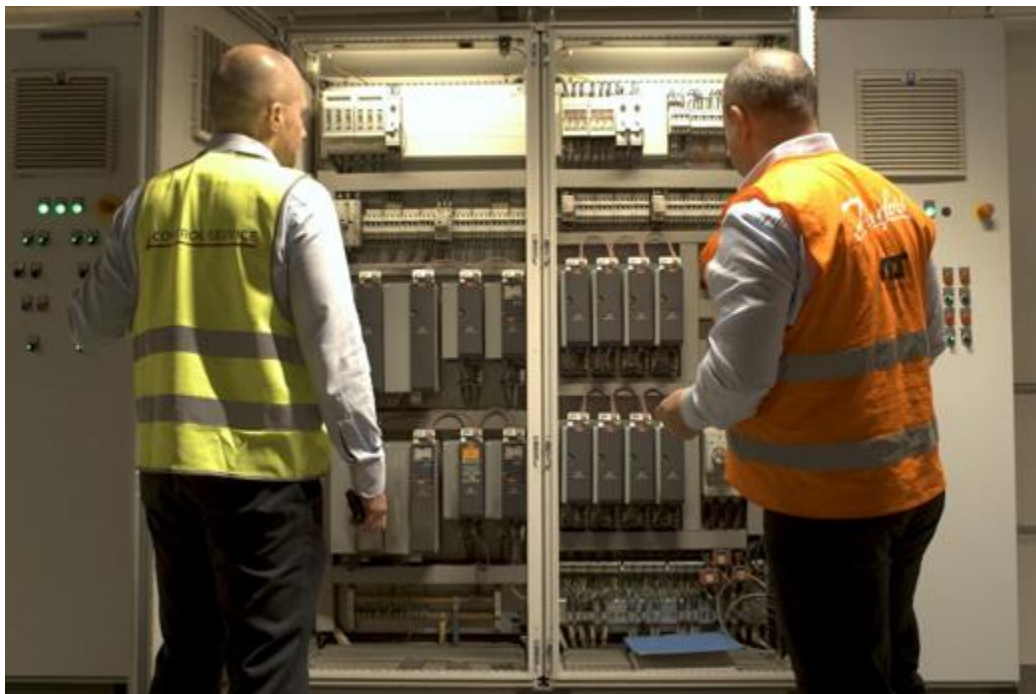
VLT® drives and soft starters optimize fan and pump control to halve the electricity bill.
